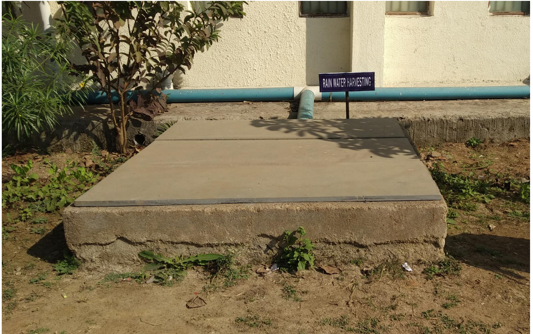
RAIN WATER HARVESTING
