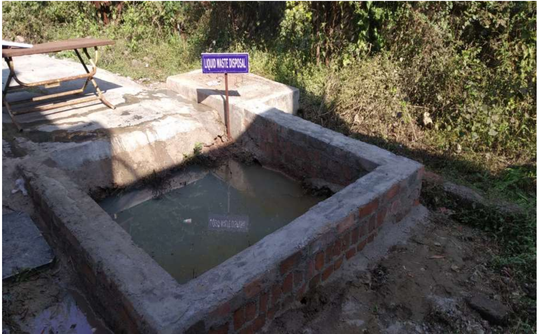
LIQUID WASTE PIT
