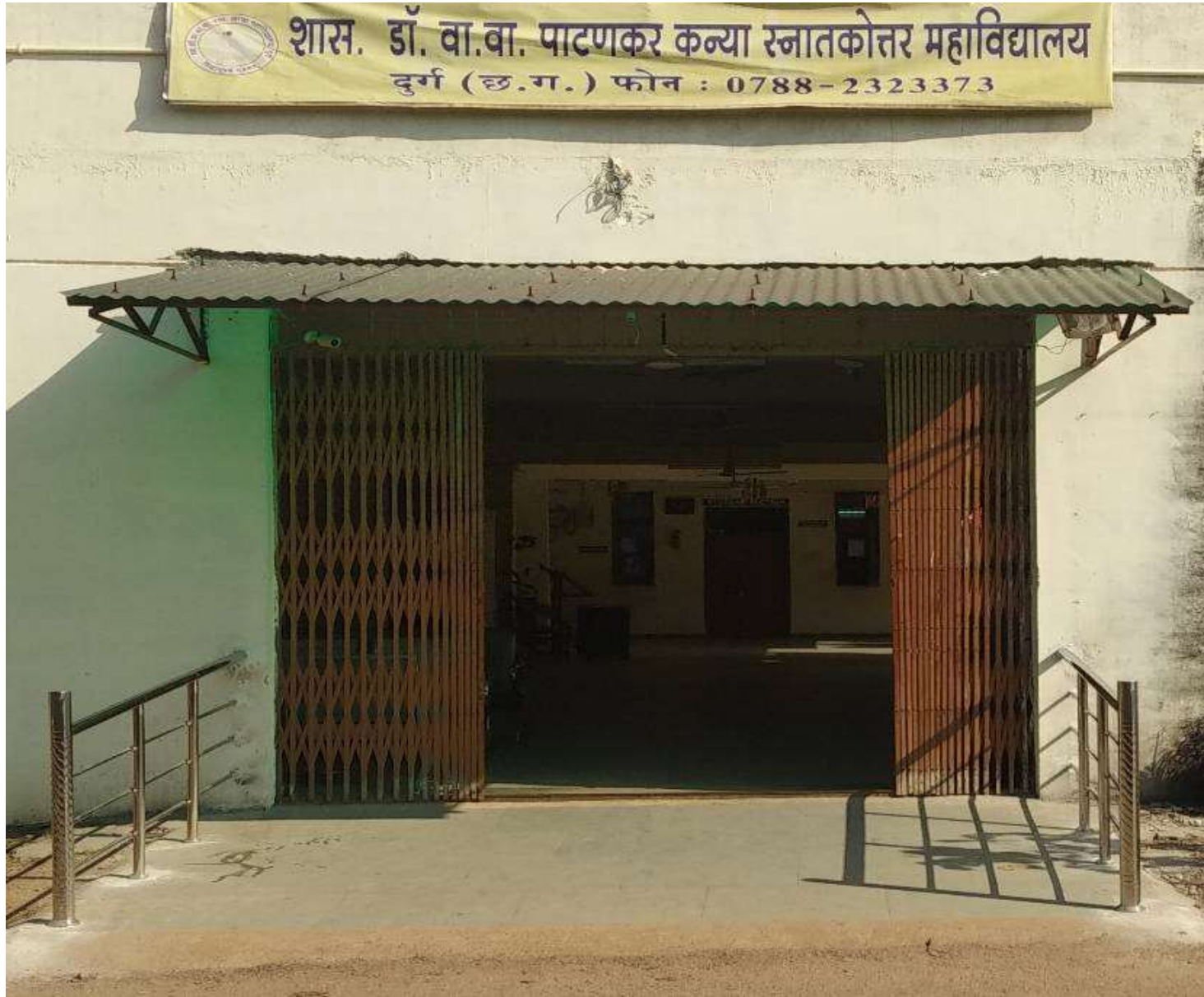
RAMP AND RAIL FOR DIVYANGJAN
