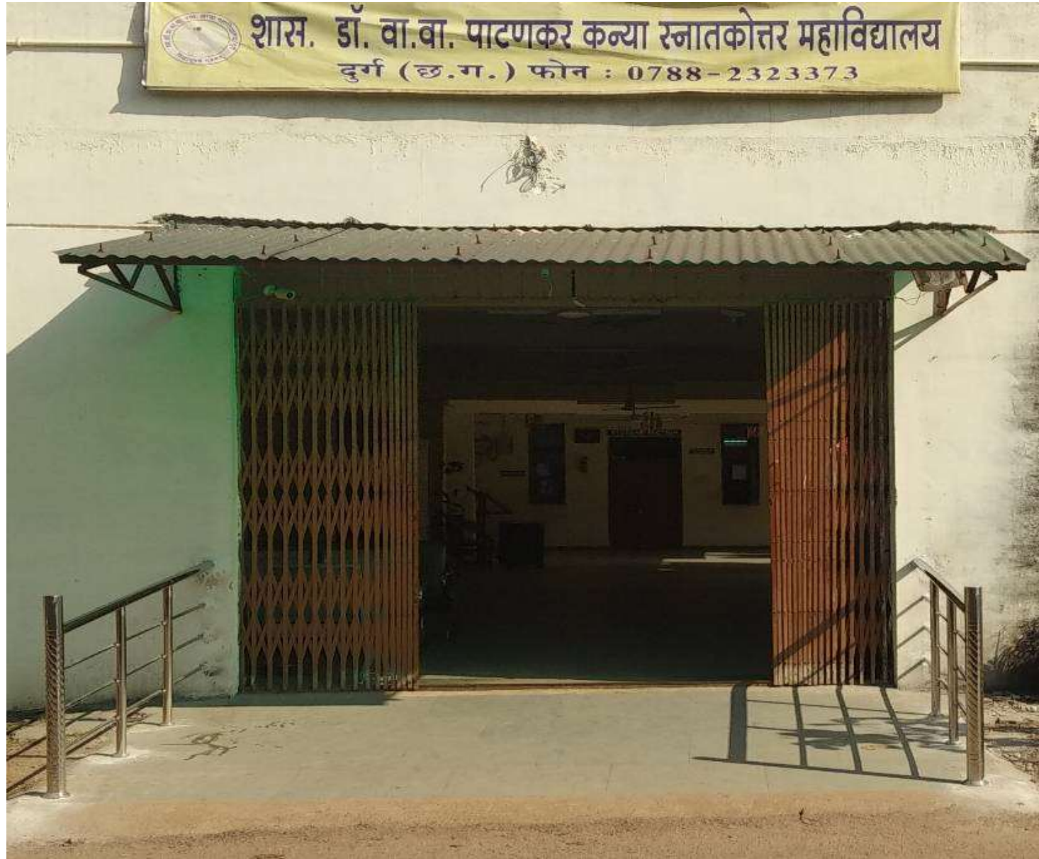
RAMP AND RAIL FOR DIVYANGJAN
