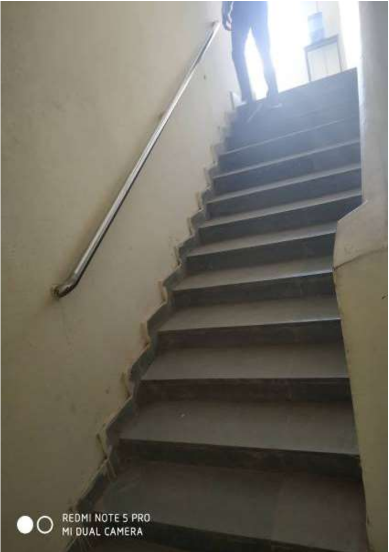
STAIRCASE WITH RAIL FOR DIVYANGJAN
